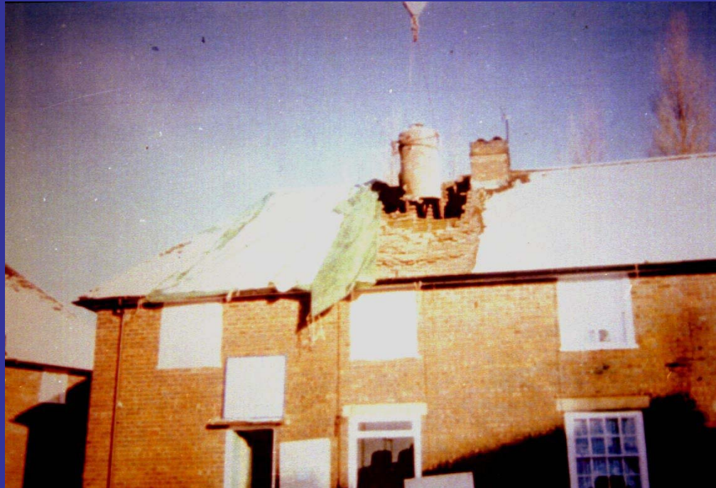
Boiler being removed from house where it landed from a factory a few hundred meters away. Cause - faulty safety valve (yield pressure of boiler about 55bar), Thanks to Philip Papard, HSE UK
