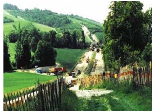
Figure 17 : cable route at site
