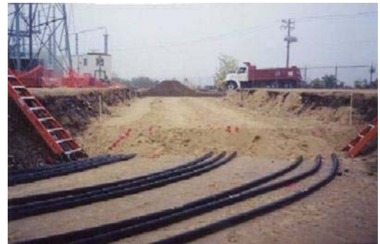
Figure 18: Installation of 400 kV XLPE cables
