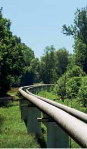
The Druzhba (friendship) pipeline system at the Czech–Slovak border. The largest crude oil pipeline network in the world, linking Russia to Germany, is among the priorities of the trans-European energy networks (TEN-E).
